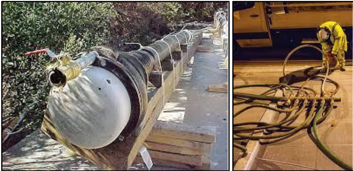
Figure (4): Vacuum grouting (Chaitanya et al., 2023).
