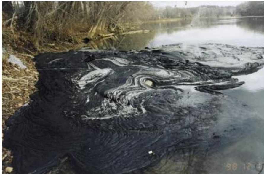
Figure (1): Hot bitumen and HMG from co-injection that escaped to the surface from deep karst.
